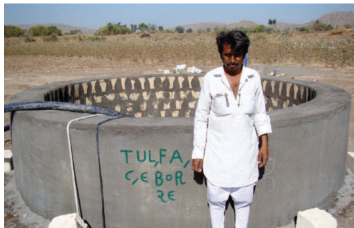
Parapet walls around wells are constructed in the Asiatic Lion Landscape to prevent accidents or wildlife falling in open wells
